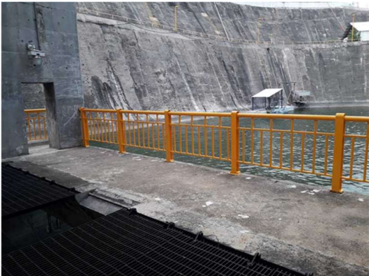
Spillway Chicoasen Dam
