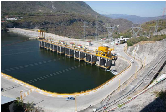
Slope protection Chicoasen Dam
