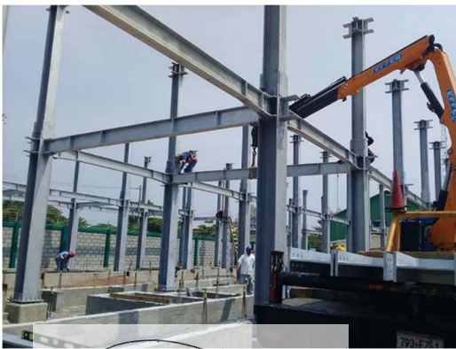
CFE office building Steel construction Oaxaca, Mexico
