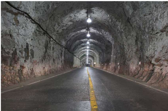
Tunnel maintenance CFE Chiapas, Mexico
