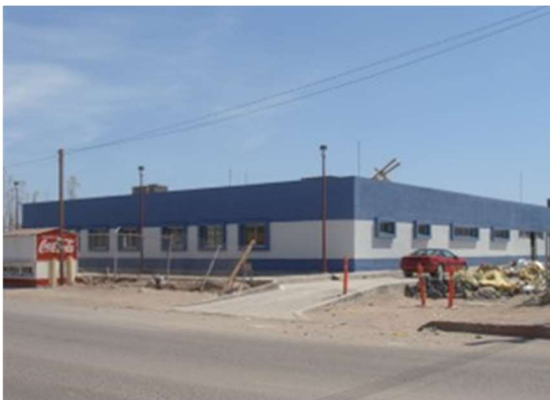
ISSSTE Hospital Cd Constitucion, BCS
