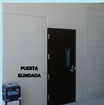
Safe room access
