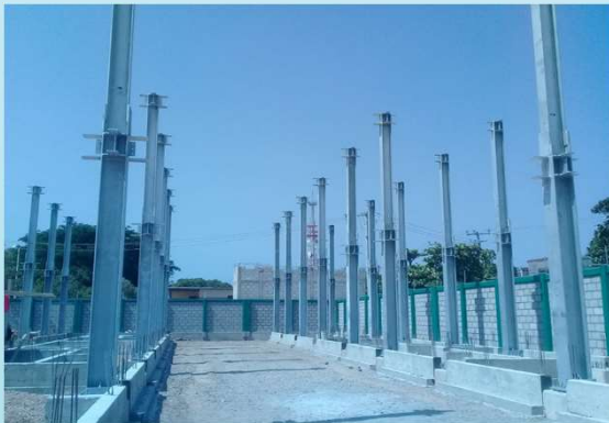
Columns fixed to foundation
