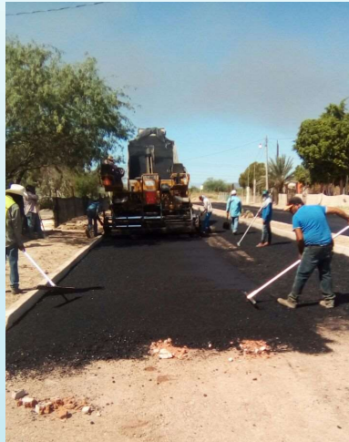
Priming prior to surfacing Road paving
