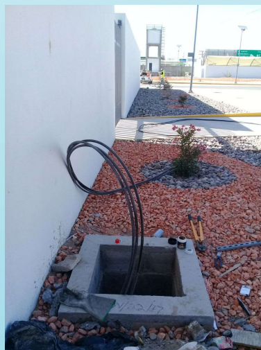
Laying underground Medium voltage installation
